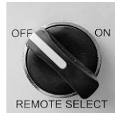
Selector Switch Switch to “OFF” when Operating from the Main Control
