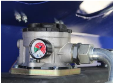
Fig 2.1. Filter Housing with Pressure Gauge
